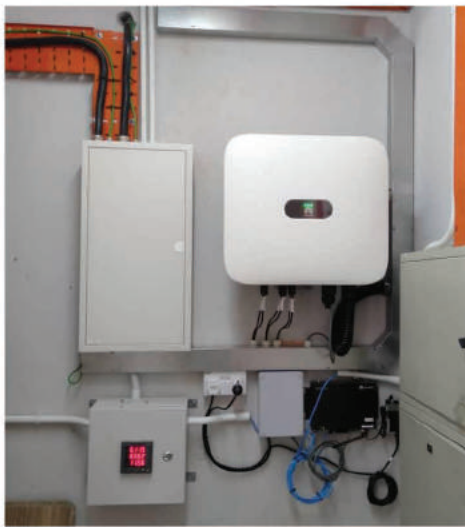
ABOVE Energy Measurement System installed in station building
