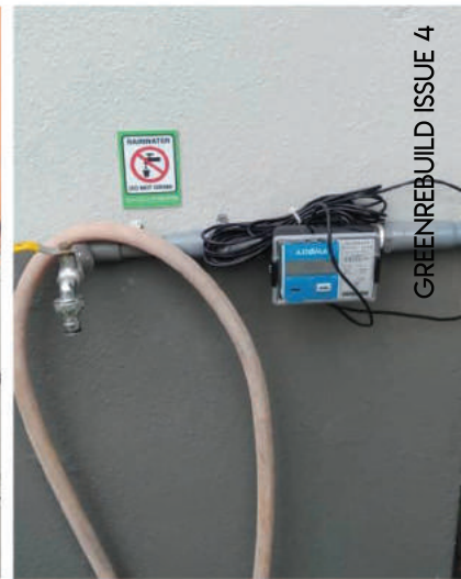
ABOVE Digital water meter installed to monitor rainwater harvested
